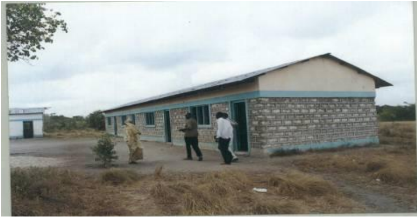
Infrastructure improvement one of wokike's strategies to improve education.
